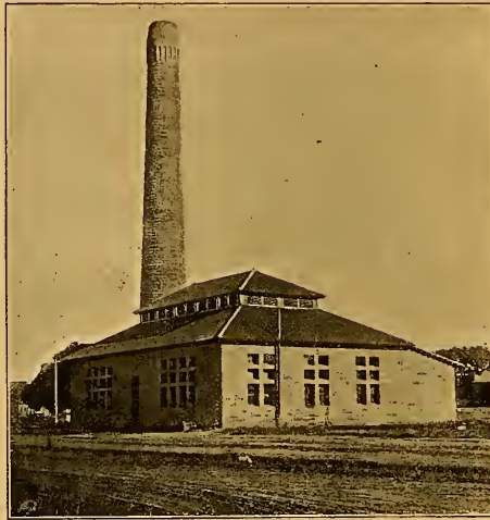
FIG. 68. POWER HOUSE, LELAND STANFORD UNIVERSITY.
